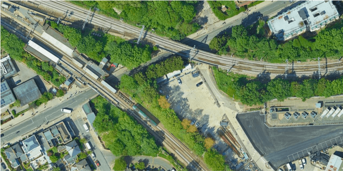
Figure 5. An example of skew bridge construction adopted by Gregory [35] near Gospel Oak station, a ward adjacent to Kentish Town in the London Borough of Camden, United Kingdom. The railway tracks heading in the northeast and southeast directions are the Suffragette (heading to Barking) and Mildmay (heading to Stratford) Overgrounds, respectively. The road beneath them is Gordon House Road. Figure courtesy of Google Maps .
