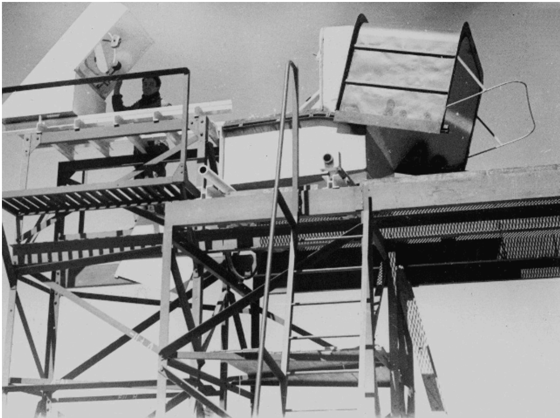
Figure 4. Detail of the first coelostat (two flat mirrors of 0.5 and 0.4 m diameter). Courtesy OP.
